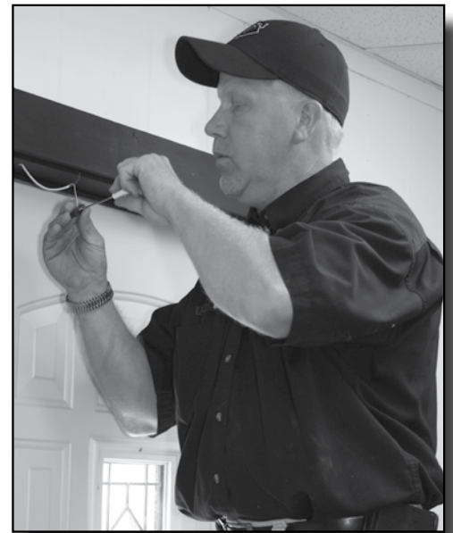
Understanding the difference between hardwired and wireless can help you better maintain your alarm system.
